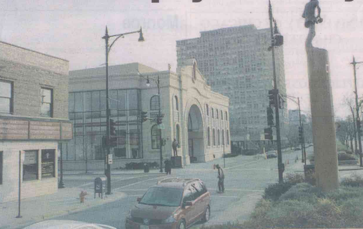
The majority of 3rd Ward Ald. Dorothy Tillman's discretionary spending for infrastructure improvements have been concentrated around the intersection of 47th Street and King Drive. Marc Monaghan
